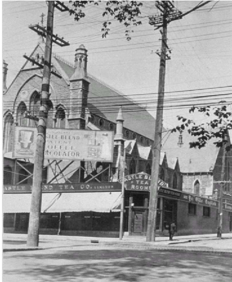
Figure 4: The Original Emmanuel Congregational Church Being Transformed into Shops, 1911 (Bibliothèque Nationale du Québec, Massicotte Collection. The original source of this image is unknown. A similar photograph appears in the Montreal Witness , 16 March 1912).
